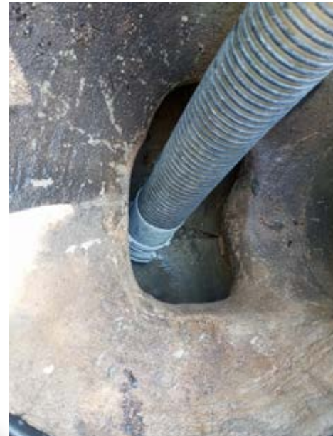
Intervention d'hydrocurage - Graveson
